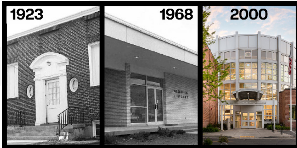
Photos showing the progression of the American Fork Library buildings over the years
